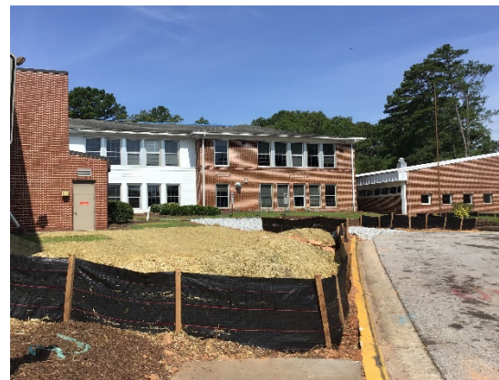
Main Entrance Erosion Control
