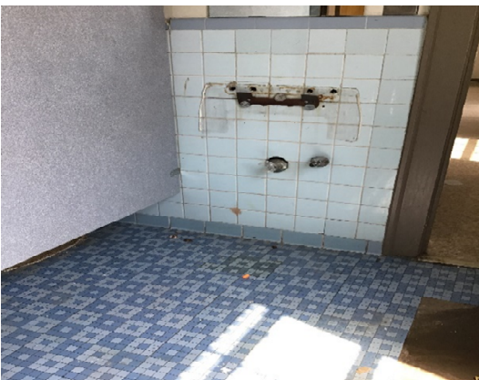
Bathroom Plumbing Fixture Removal
